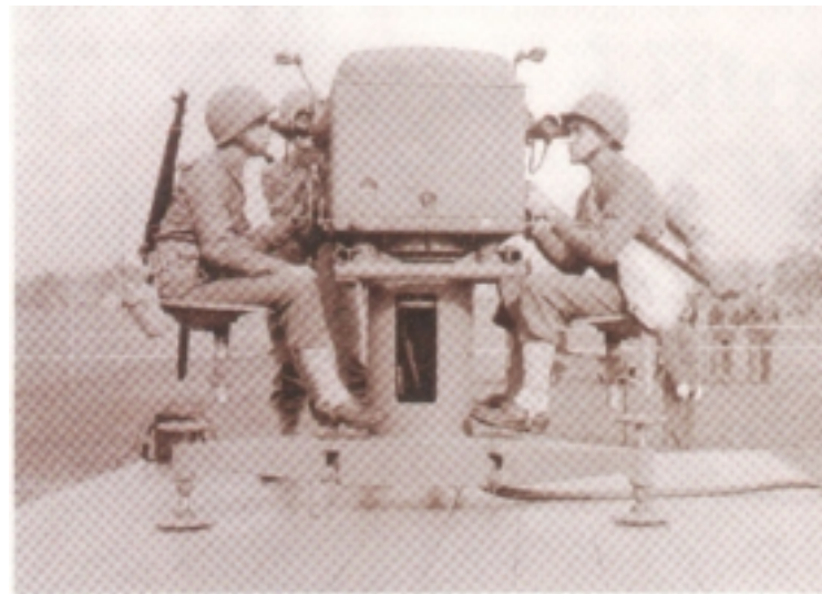
The tracker of the M-9 electrical gun director in action. As one soldier orients the telescopes in elevation, the other orients them in azimuth by turning the entire tracker head.
